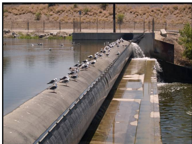
Rubber Dams are an Effective and Environmentally Friendly Means to Temporarily Block River Flows to Induce Groundwater Recharge
