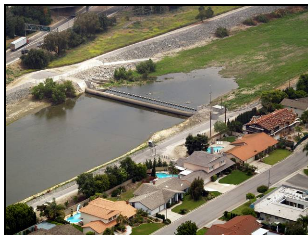
Rubber Dams are an Effective and Environmentally Friendly Means to Temporarily Block River Flows to Induce Groundwater Recharge
