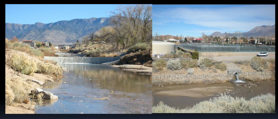
The Bear Canyon Recharge Demonstration Project was designed to recharge surface water to the Middle Rio Grande Basin aquifer through an instream infiltration system along the Bear Canyon Arroyo in northeast Albuquerque.
