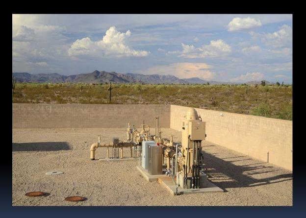
The first ASR well in the United States to incorporate the "reverse-siphon" injection method and deliver recovered supplies directly into the distribution system. Operates at 2.6 MGD (10K m<sup>3</sup>/day)
