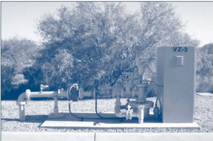
A reclaimed water recharge well in Phoenix, AZ. SOURCE: Andy Terrey, City of Phoenix.
