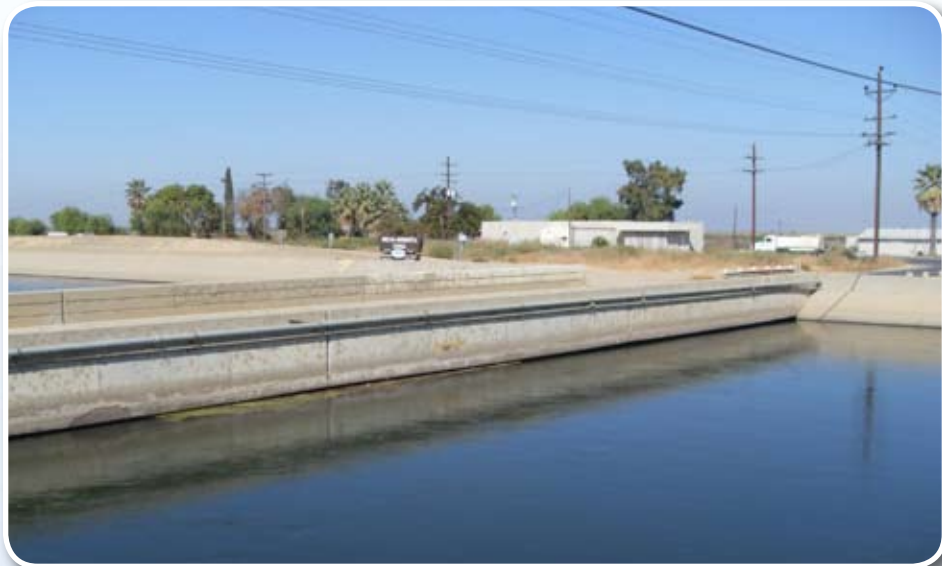
Figure 2. Reduced Canal Freeboard in the Delta Mendota Canal Downstream of Check 18 due to Subsidence (Source: Central California Irrigation District)
