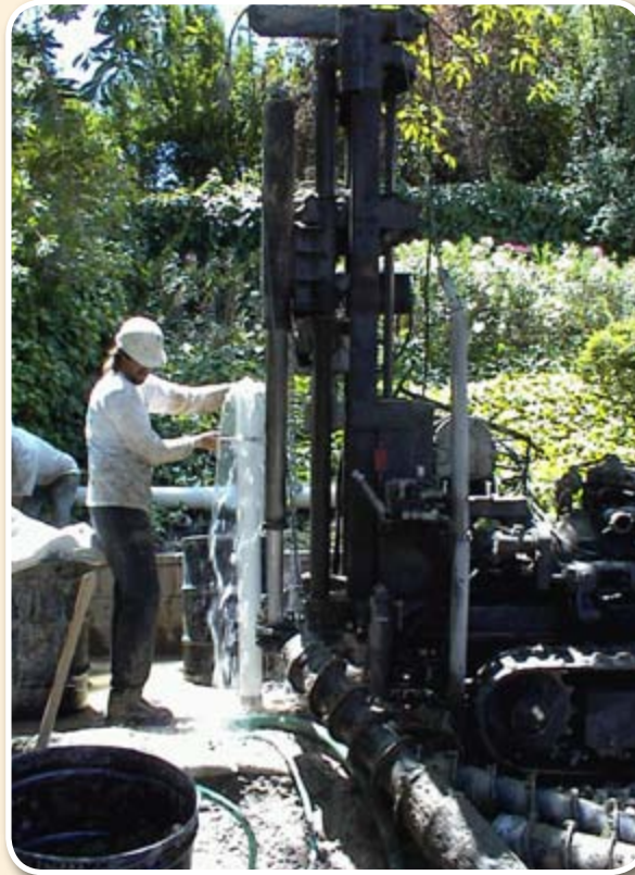
Figure 1: Track-mounted Hollow Stem Auger drilling rig installing a 15-foot deep by 4-inch \phi flowing artesian dewatering well in a residential subdivision of Pleasanton, CA, circa 1998. The track-mounted rig allows for access in rugged and small areas that larger truck-mounted rigs could not negotiate and reduces the post-construction footprint. The right forefront of the picture shows three 10-inch \phi flight augers with drill cuttings still wrapped around the flightings. The well was constructed within the hollow stem of the flights prior to removal of the drill string. (Photo courtesy of E.D. Hendrix, P.G., C.Hg., Daniel B. Stephens & Associates, Inc.)
