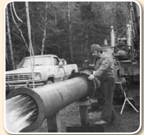
Figure 1a: Note the unique type of sounder to the right of the driller during an 8,000 gpm pumping test (drawdown of about 4 feet) circa 1976 9 .
