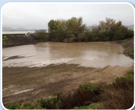
Figure 3. Infiltration basin in Pajaro Valley, CA.
