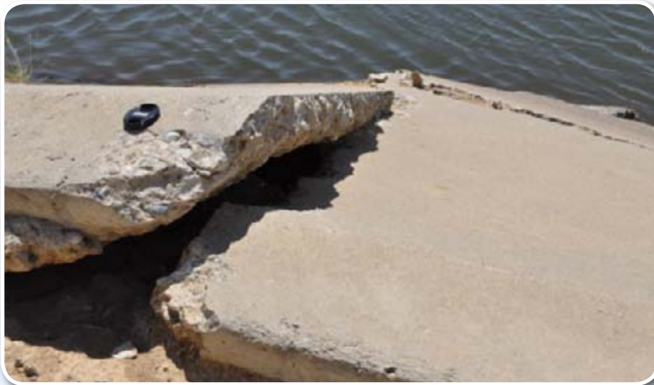
Concrete sidewall of the Delta-Mendota Canal, buckled from subsidence.
