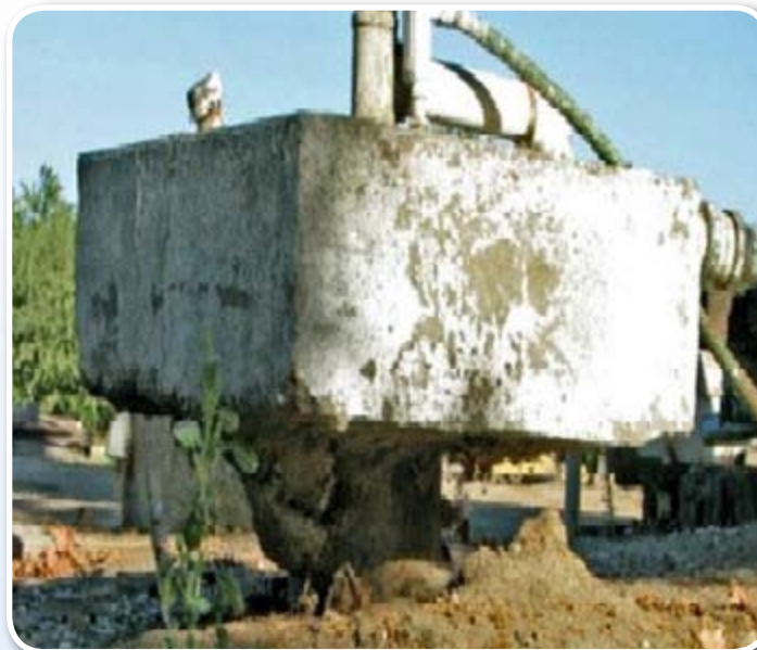
Concrete well pad, and well, exposed by land subsidence; in this case, the well is intact.
